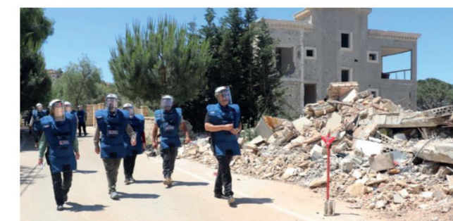
Building clearance and rubble removal task in Arnoun village, Nabatieh governorate: A race against time as people are returning quickly following the attacks.
