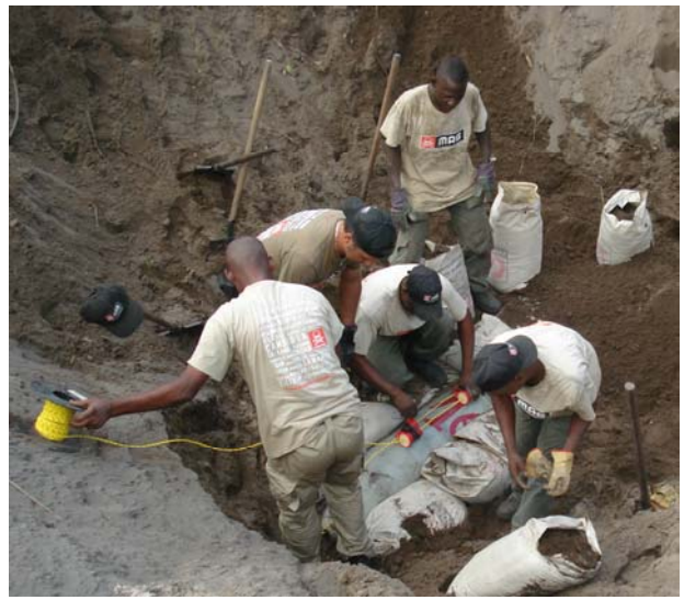
Rigging an OFAB 500 (HE) for controlled demolition
