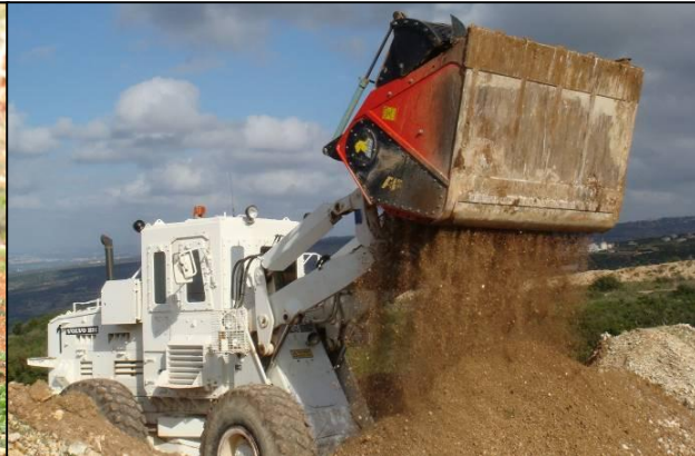
MAG's armoured Volvo working on the Blue Line
