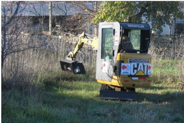
Mechanical vegetation cutting using mini excavator with flail
