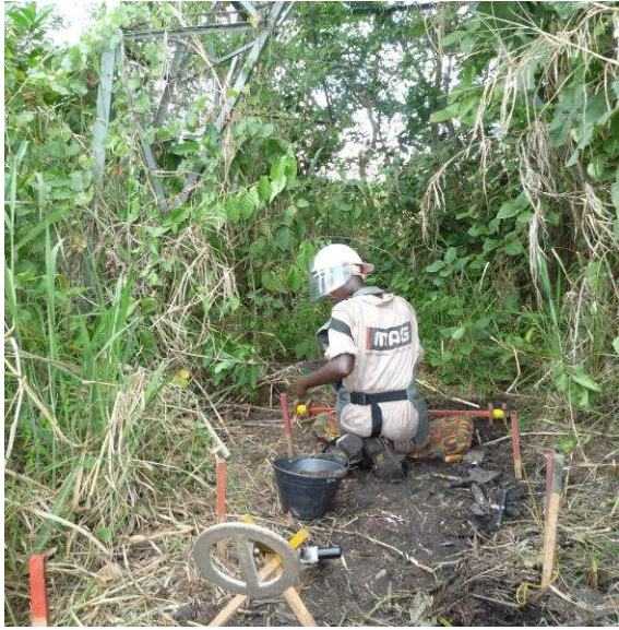
Manual clearance around an electric pylon
