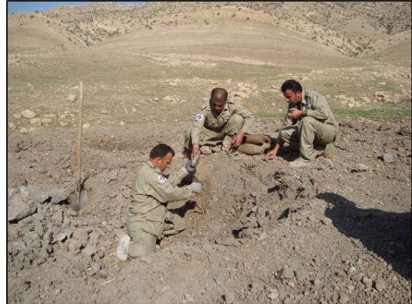
CWMD team preparing for demolition of hazardous items in Chamchamal, Sulimaniyah
