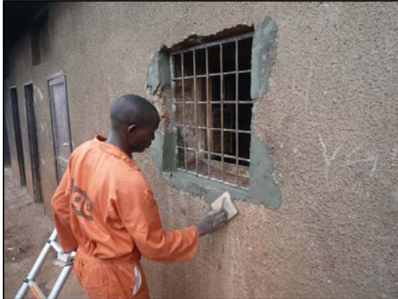
A member of the MAG Physical Security team secures the window of Muyinga's police station, Police Region East
