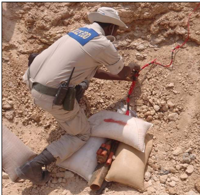
Somalia: EOD Team Leader sets up small multi item demolition in Garowe
