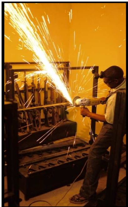
Somalia: Police armoury construction
